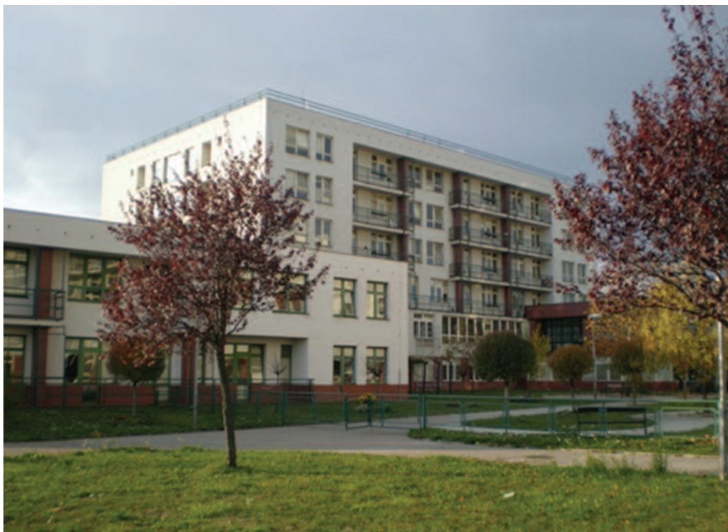
Photo no.1: The main building of the facility for seniors Věstonická 137
