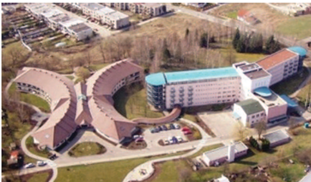
Photo no. 7: Facility Domov U Biřičky 144
